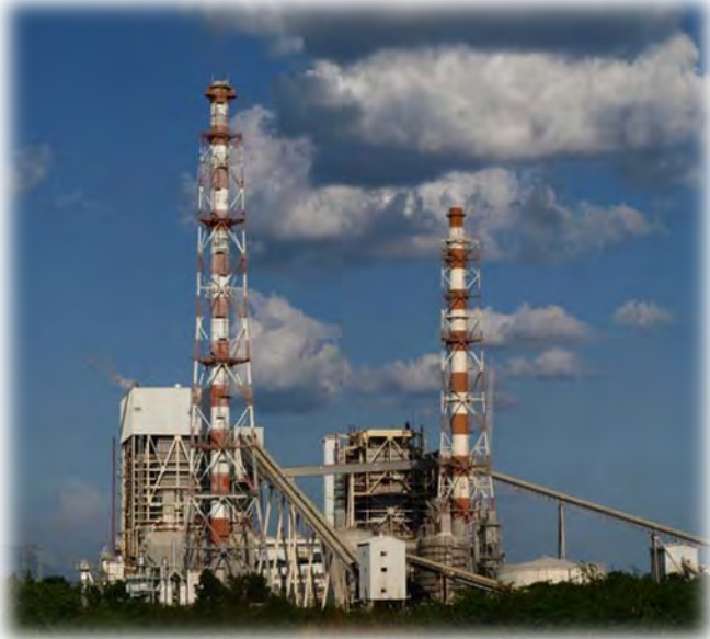
600MW Coal-Fired Power Plant Calaca, Batangas
